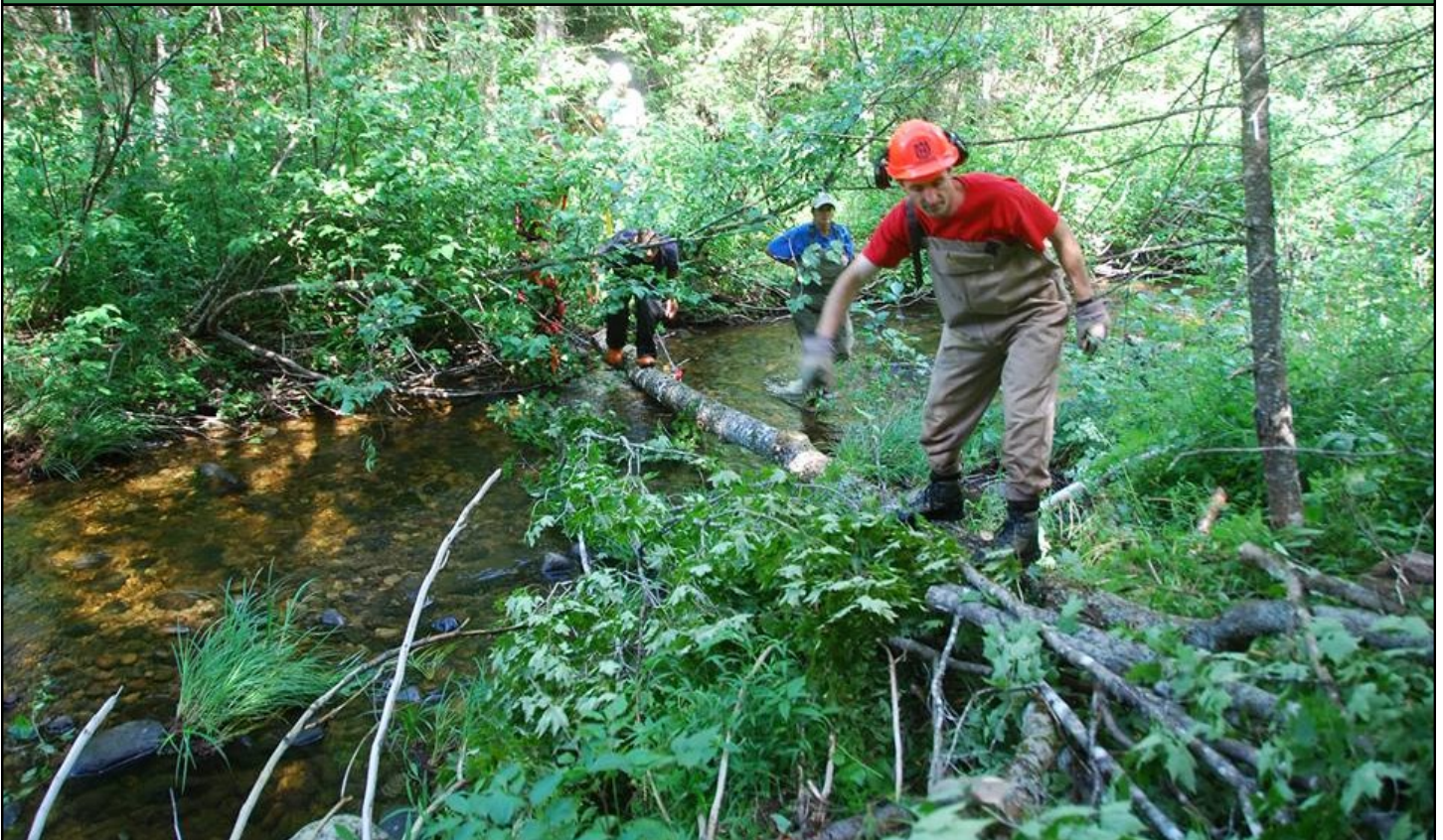
Improvements being made to existing trout habitat. Photo courtesy of Vermont Fish & Wildlife
